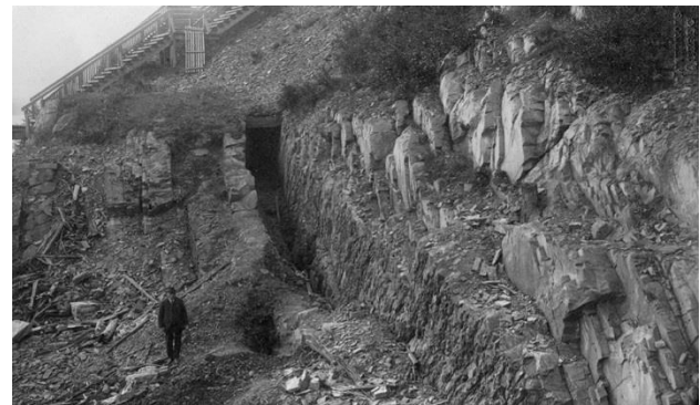
Figure 8. Example of one of the large fissures (fissure A located in Figs. 7 and 9) mapped by Baillargé in 1879 and partly filled by debris. Note the wood cover near the top. Photograph likely taken while the slope was being repaired after the 1889 slide. (Source: archive of the City of Québec).
